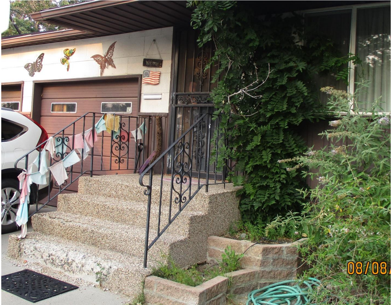
(View of front steps of 630 Lester Avenue)
